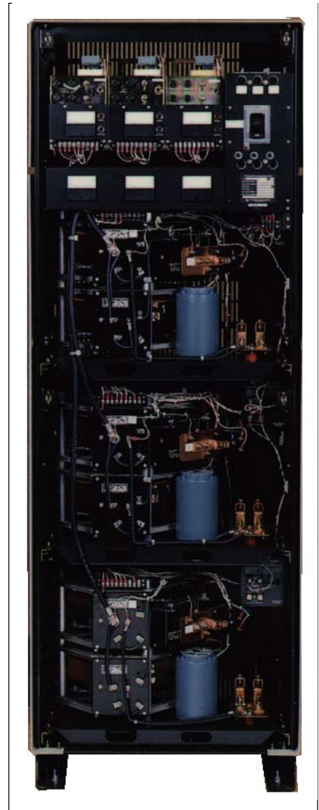
Unit shown is a 3 phase, 108 kVA regulator with individual phase control, circuit breaker, and ammeters.
