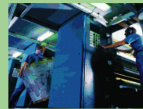
Process & Control Equipment
